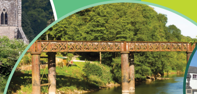
Viaduct at Redbrook
